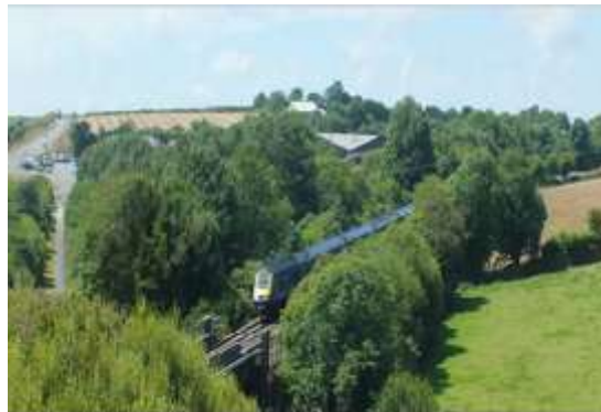
Mainline railway at Treburgie Water
