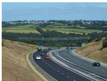
Dobwalls A38 Bypass
